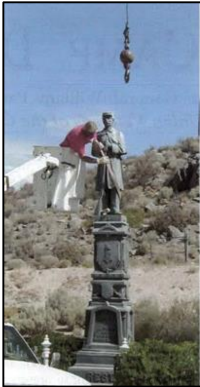
Crew Removes Top Section
